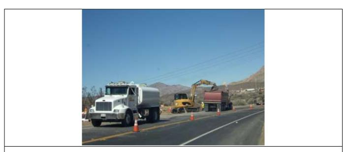
**Photo 3:** Water trucks were on site to suppress dust emissions during curb work at SP-91 in compliance with MM-BIO-4a and MM-AQ-1.
