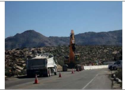
**Photo 2:** In accordance with MM-BIO-4a and MM-AQ-1, crews were observed covering spoil loads leaving Section 3 of the underground alignment.
